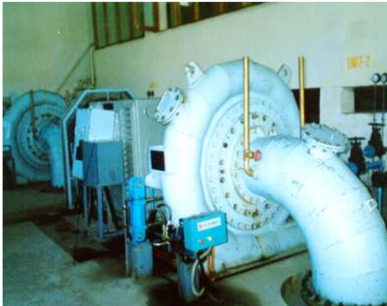
Solang HEP 3 X 500 kW ,Horizontal Francis Turbine
