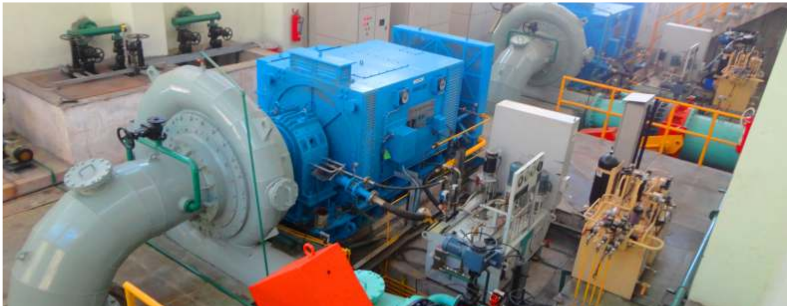
Sechi HEP 2X2.25MW , Horizontal Francis Turbine
