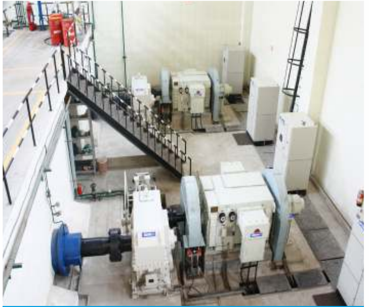
Ranni Perunad HEP( Gearbox-generator Assembly) 2 X 2 MW ,Horizontal Kaplan Turbine
