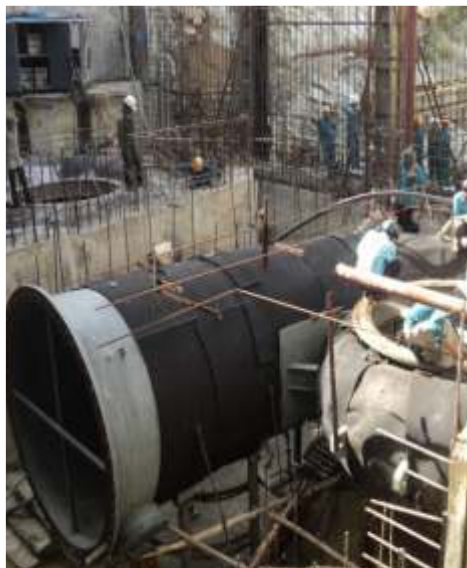
Erection of Spiral Casing
