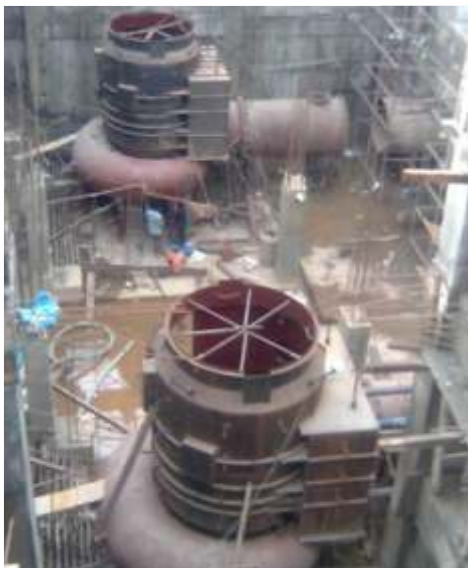
Erection of Spiral Casing & Pit Liner
