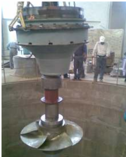
Erection of Vertical Kaplan Runner Assembly at Site.
