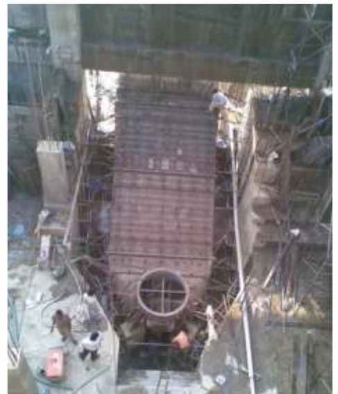
Erection of Draft Tube
