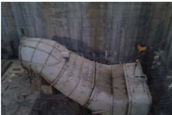
Erection of Draft Tube
