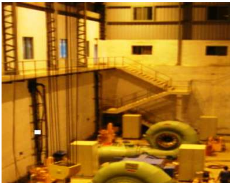
Aniyur HEP 2 X 3 MW ,Horizontal Francis Turbine
