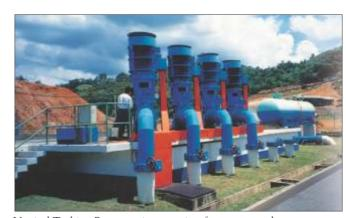
Vertical Turbine Pumpsets in operation for water supply scheme at Sabah, East Malaysia
